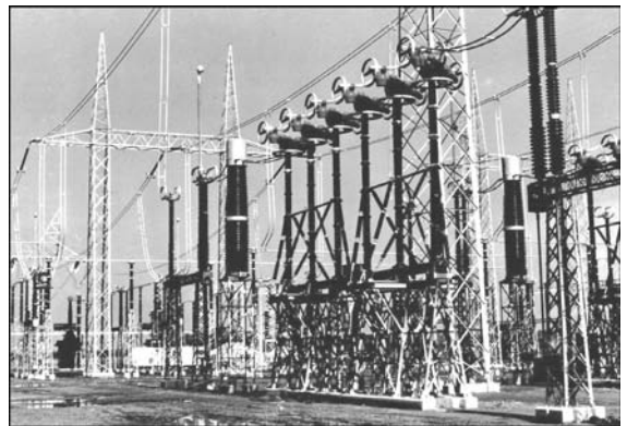
Figure 2 Air-blast circuit breaker type PK12 applied to 765 kV in North America (Courtesy of Alstom Grid)
