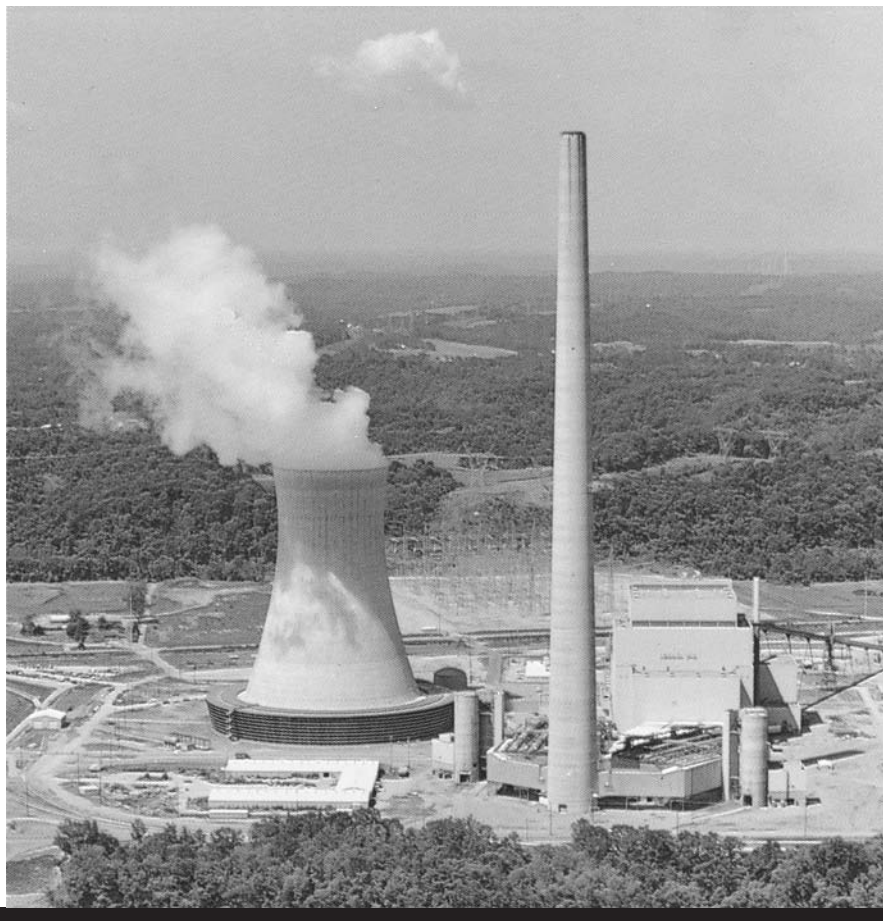
1300 MW coal-fired power plant (Courtesy of American Electric Power Company)
